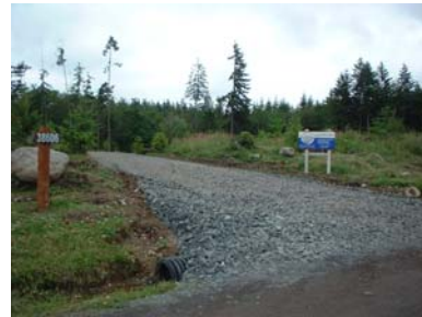
Left Good example of a culvert installation
