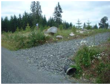
Left Good example of a culvert installation
