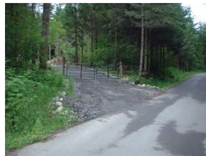
Right & Left These driveways will allow rain water to run into the adjacent roadway rather than the ditch line
